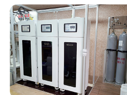
- Dongsong Sewage Treatment Plant in Cheorwon city
