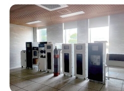
- Chilbo Water Purification Plant in K-water
